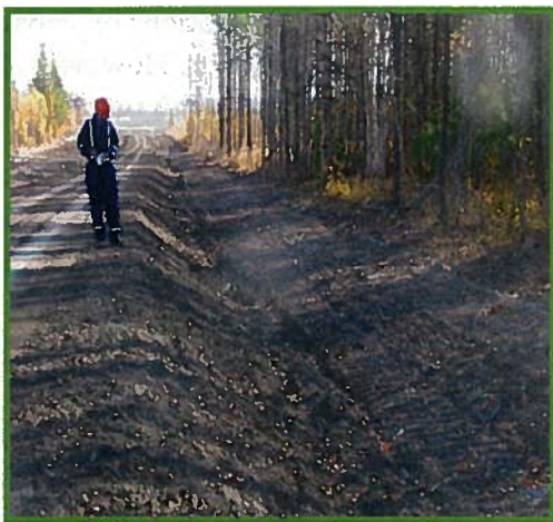
No stockpiled soil along access road.
