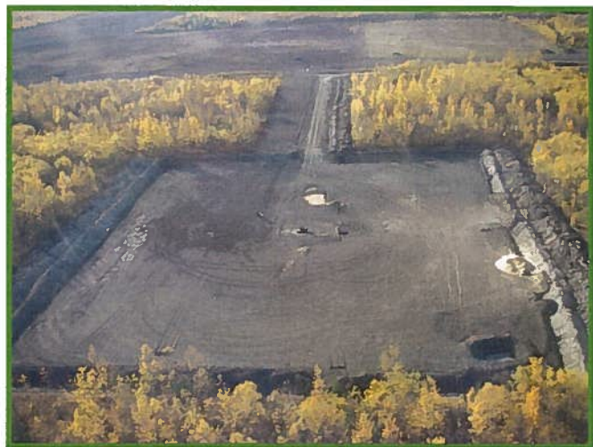
Good separation of topsoil and subsoil around well site, and along access road. The soil stockpiles have not yet been seeded.
