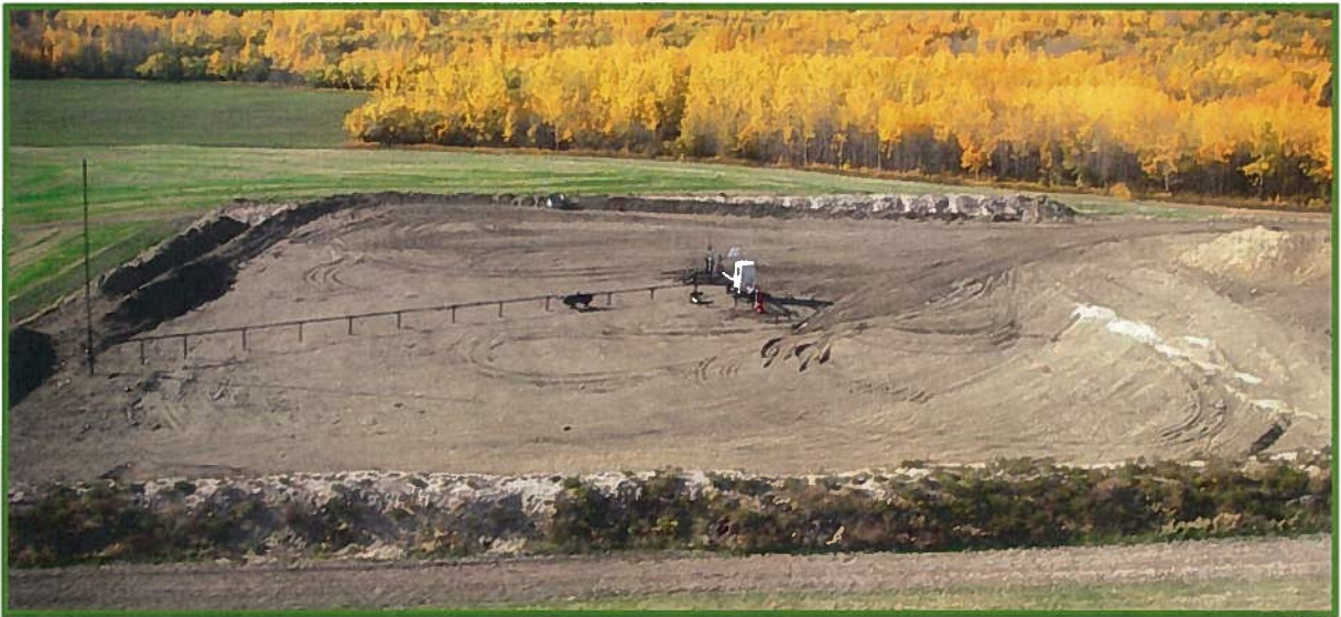
Stockpiled soil without adequate seeding –weed infestation noted in foreground.
